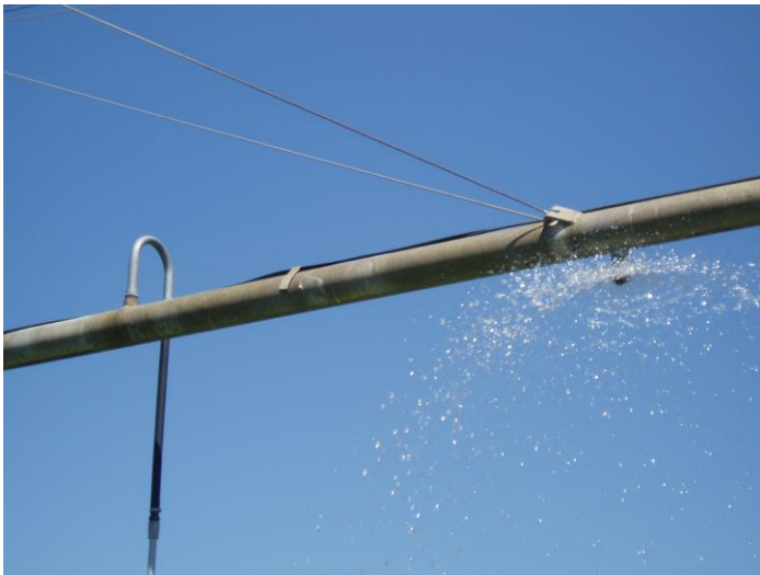
Valve leaking.
