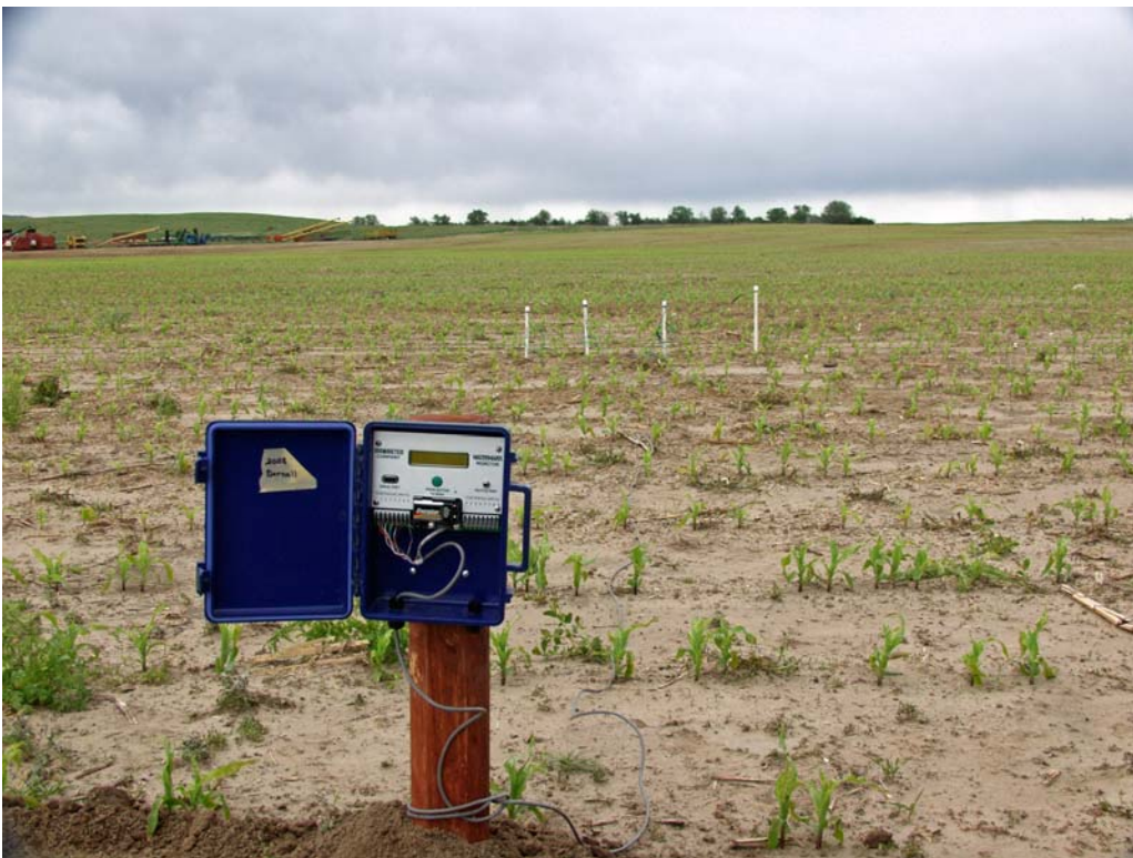
Figure 11. WaterMark™ Soil Moisture Sensor Field Installation.
