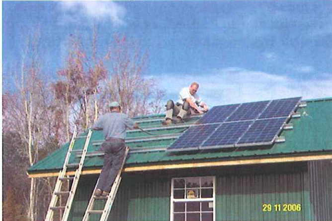
Installation of solar panels
