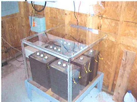
Battery Bank – Covered and vented
