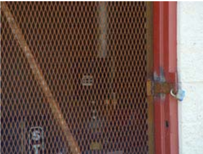
Metal Screen Door for Airflow/Vandals
