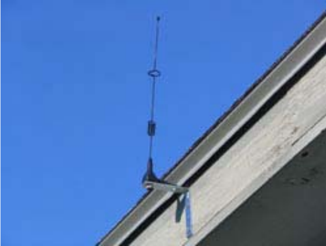
Antenna Mounted on Pump House Roof
