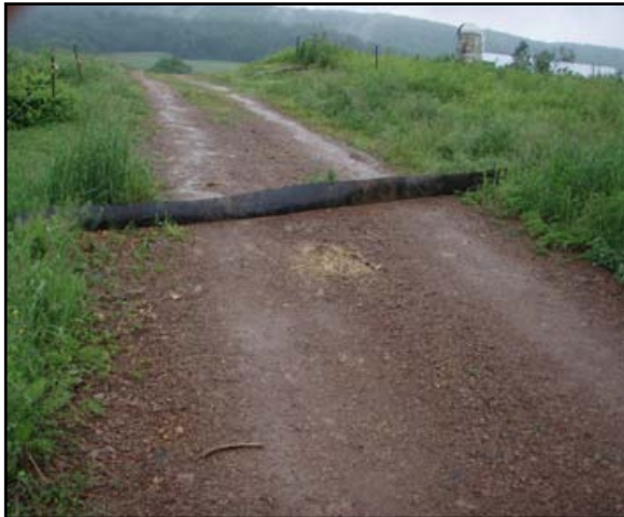
Completed Conveyor Belt Diversion
