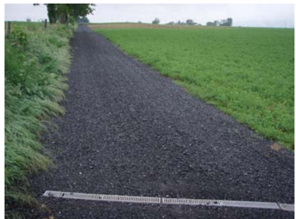
Figure 4.7: 2009 image of the improved Stuck Farm Lane.
