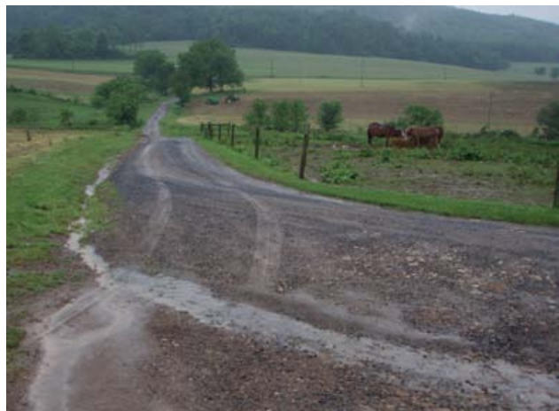
Figure 1.1: Many farm lanes act as conduits for sediment and nutrient runoff from nearby agricultural fields to streams.
