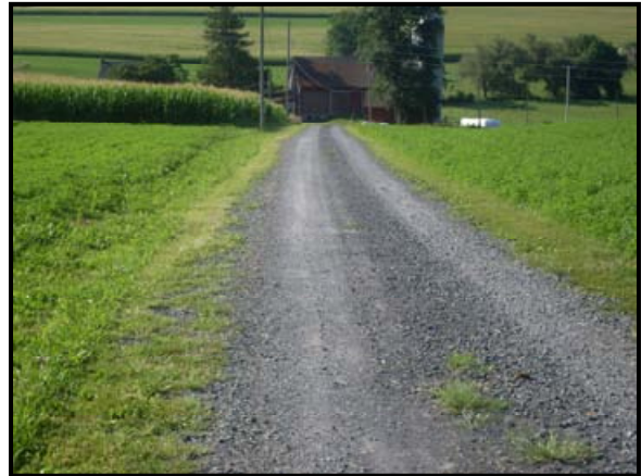
Figure 4.3: 2009 image of Yoder Farm lane and grass-lined swale.
