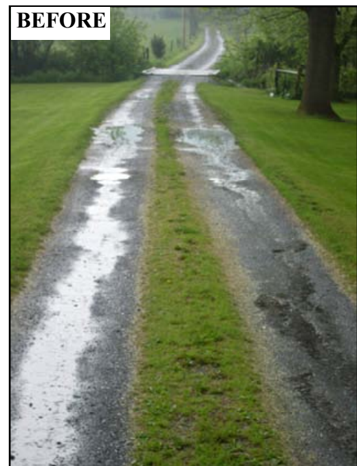
Figure 4.19: The existing lane just before construction carries water in the wheeltracks to the bridge in the distance.
