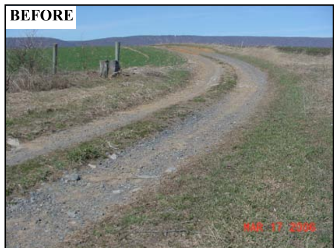
Figure 4.8: The existing farm lane with incised wheel tracks.
