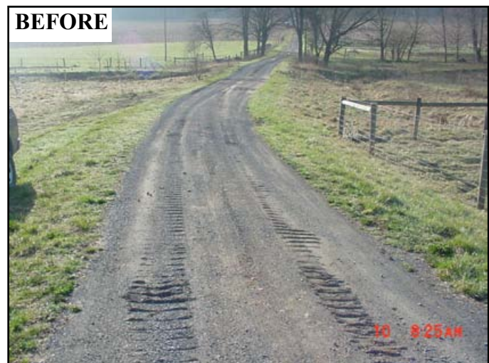
Figure 4.15: The existing lane just before construction.
