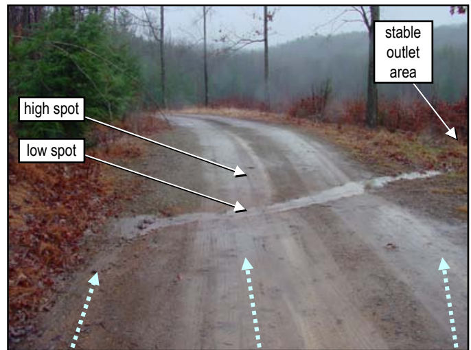
This broad based dip in Huntingdon County is located on an access road that is only open to the public for hunting season. This low-use road is ideal for broad based dips instead of crosspipes to reduce long term maintenance. The dip pictured here collects road and ditch water and directs it from left to right across the road.
