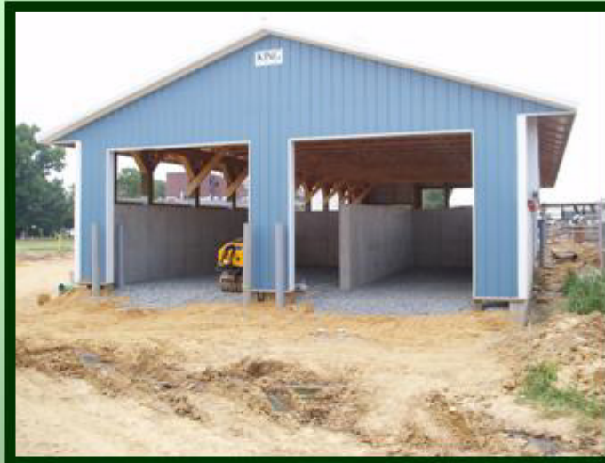
Pole Barn Construction
