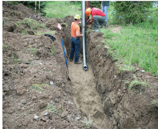
Installation of conduit from pole
