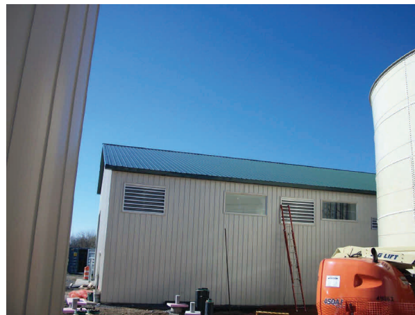
Generator room louvers—outside
