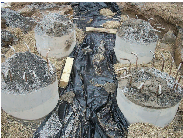
B251 Tank Foundation—Flowable Fill Cover
