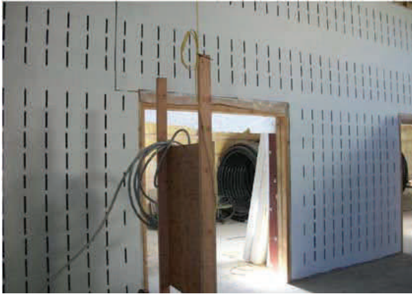
Walls in the Main Building
