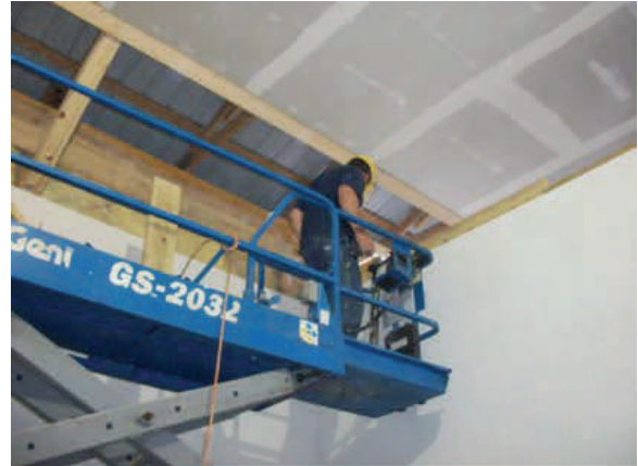
Painting Ceiling in Main Building
