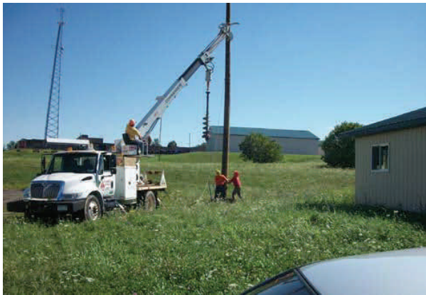
Installation of poles for the high voltage line
