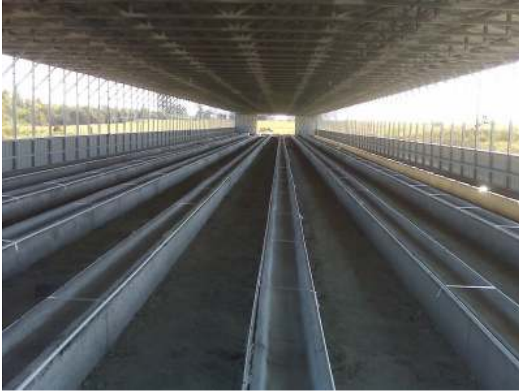
Vermicomposting Barn and Trenches.
