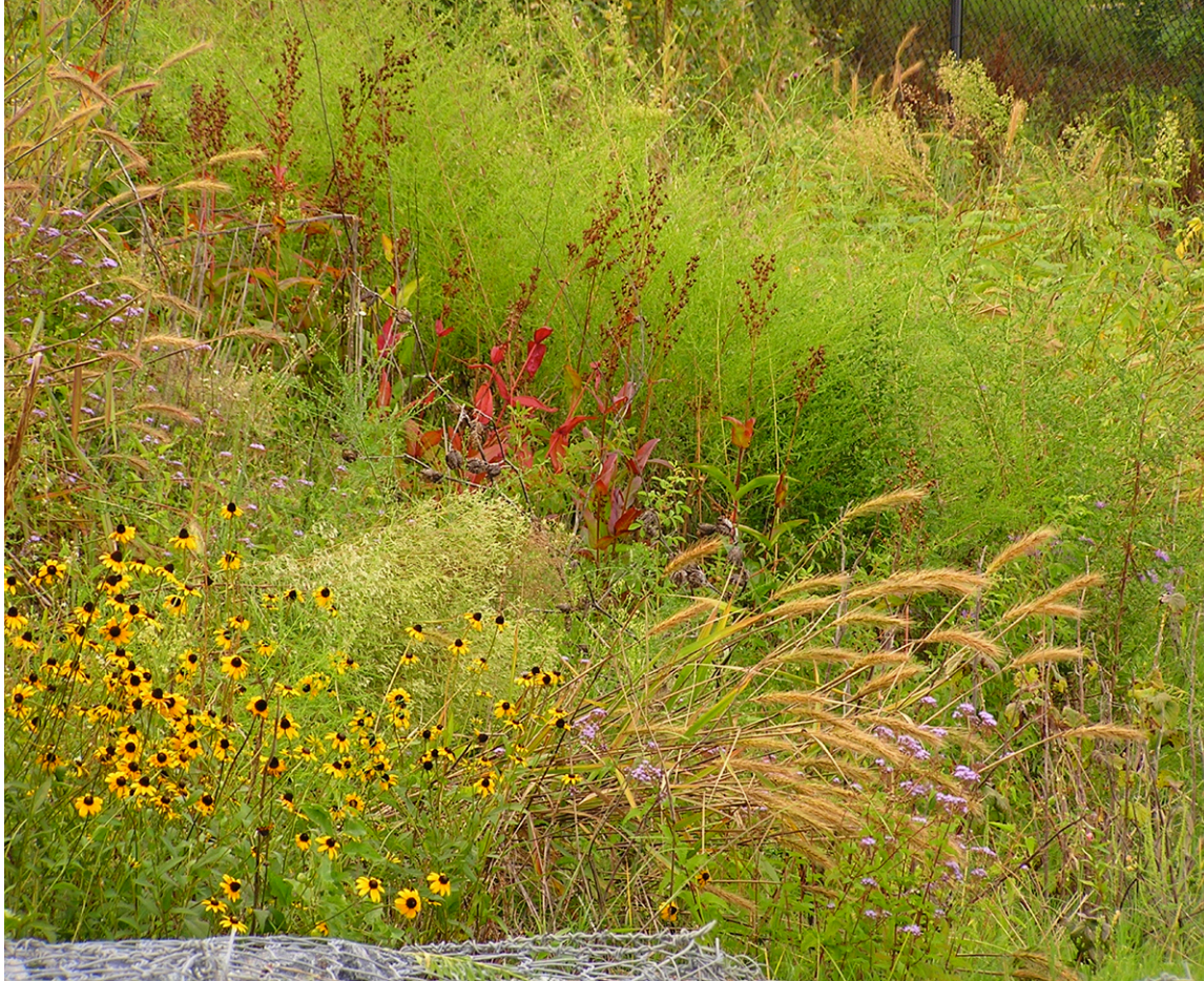
Figure 4. Successfully Stabilized Cut Slope.
