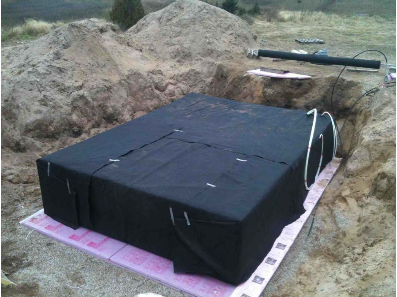
Figure 1.2 Completed and wrapped irrigation container prior to backfilling
