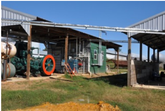
Engine (with red/green wheel) which will be connected to the electrical generator
