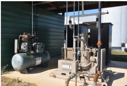
Scrubbed gas compressor (capable of 150 psi)
