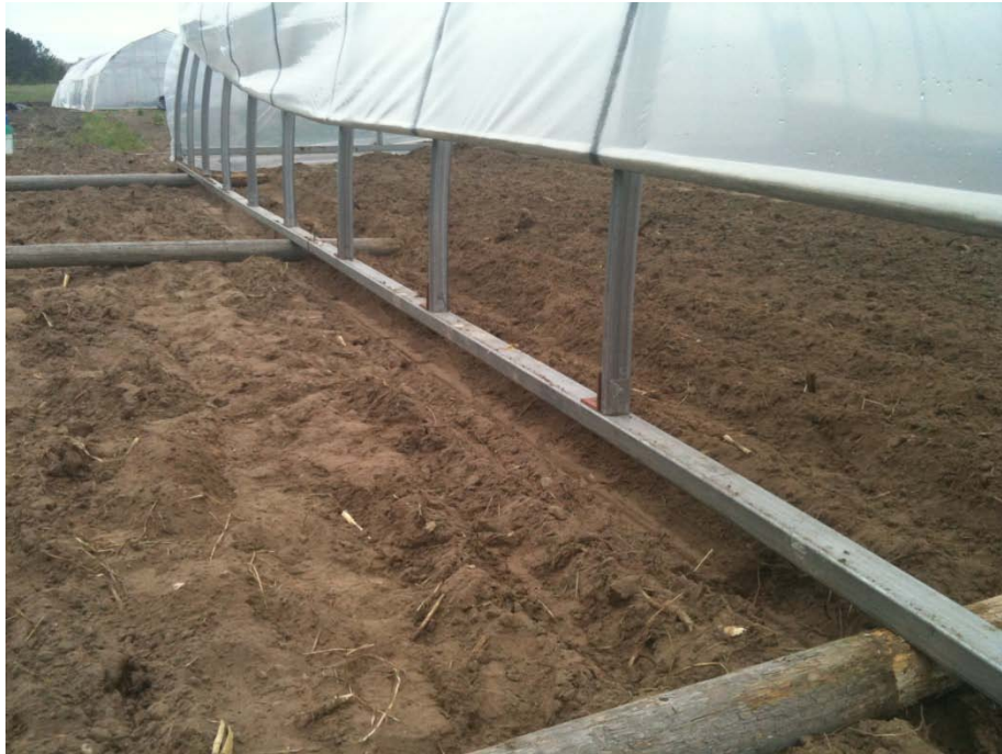
Figure D-3 Tunnel Ready for pulling to new location
