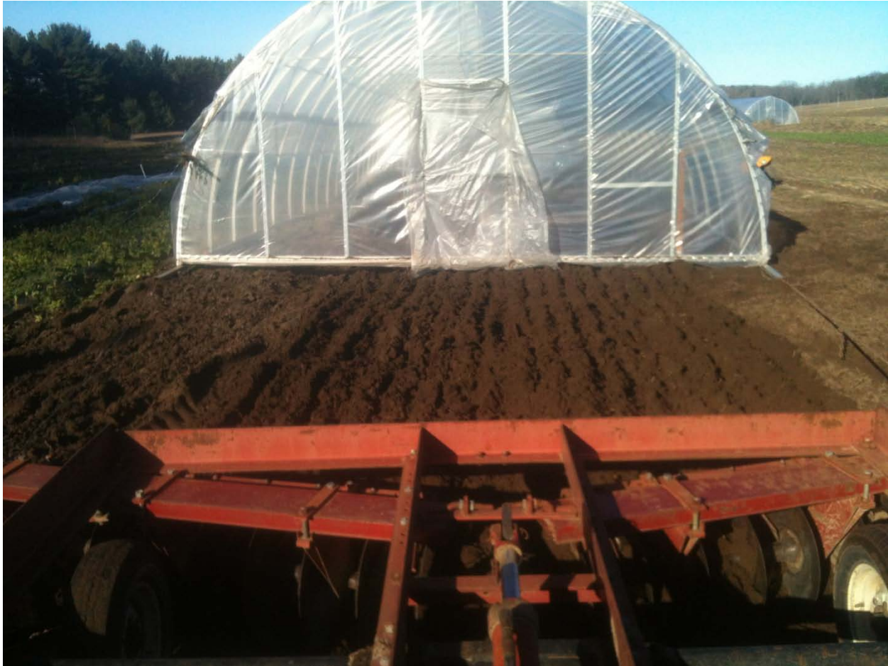
Figure D-4 Pulling a tunnel forward with a single tractor and disk
