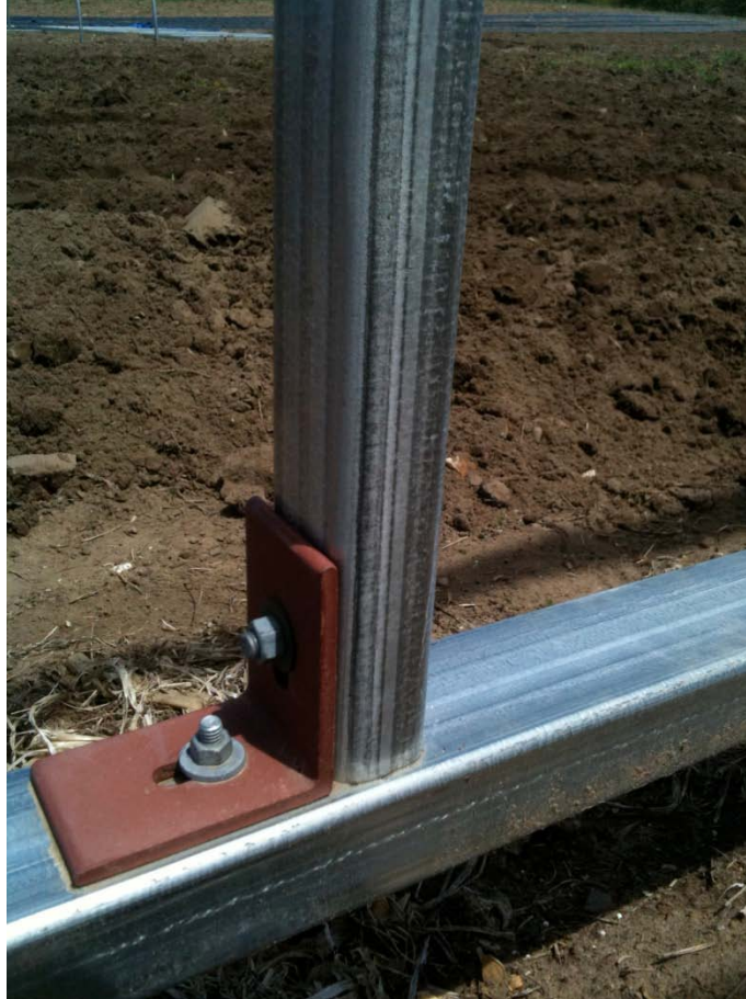
Figure D-2; Bolted angle iron attachment Bracket
