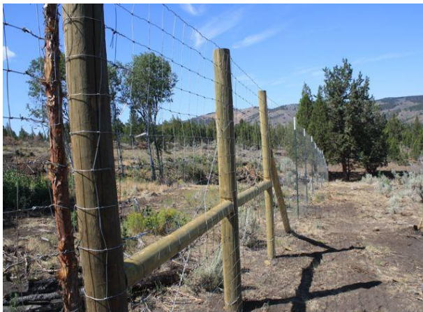
Photo 5. Woven wire big game fence constructed at the Foster demo site.
