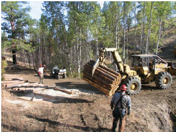
Photo 3. Buck and pole fence construction at Dovenberg demo site.
