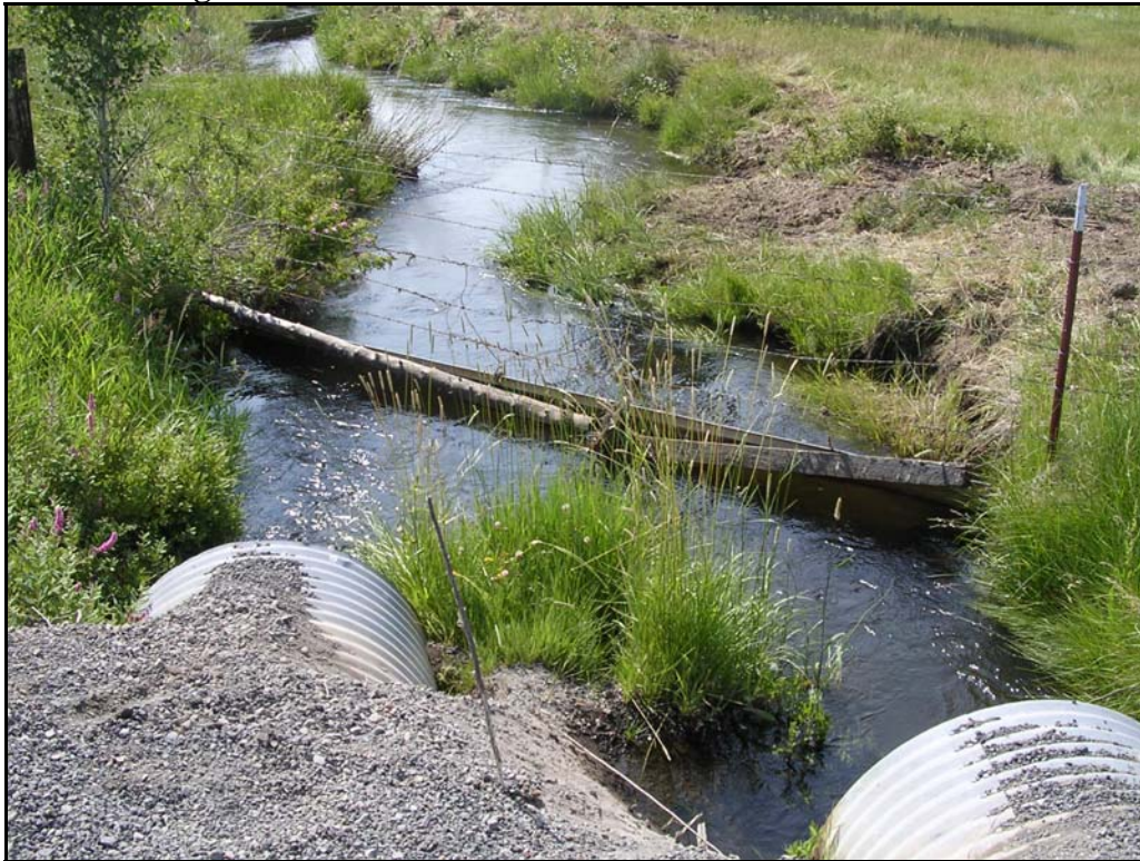
Site # 31 – looking downstream
