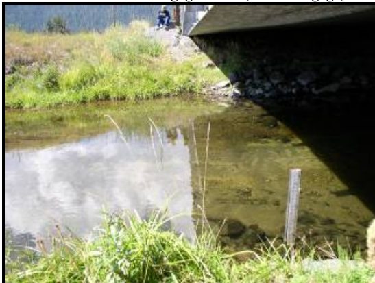
View across channel at gage section, and staff gage, LB
