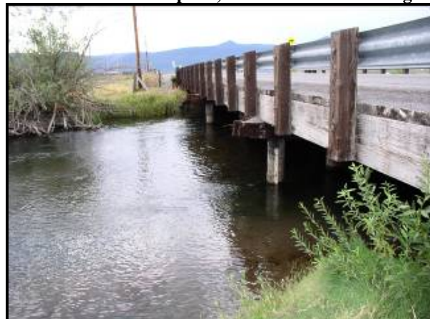
View of older staff plate, downstream side bridge
