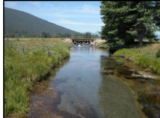
View upstream from bridge to large diversion structure
