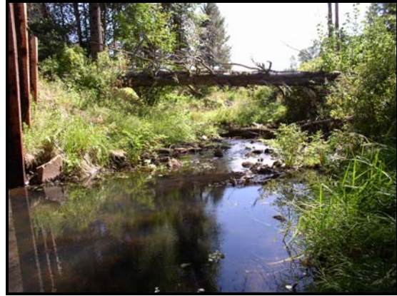
View downstream under bridge
