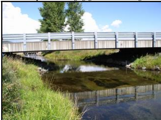
View upstream through gage section and bridge
