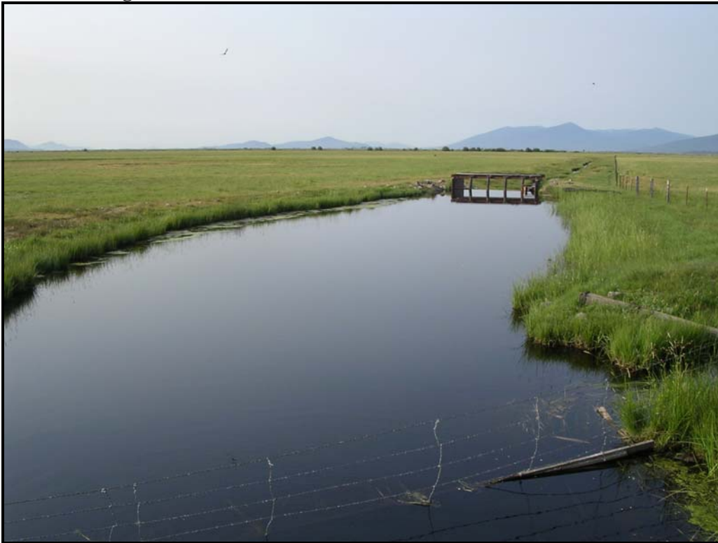
Site # 29 – looking downstream
