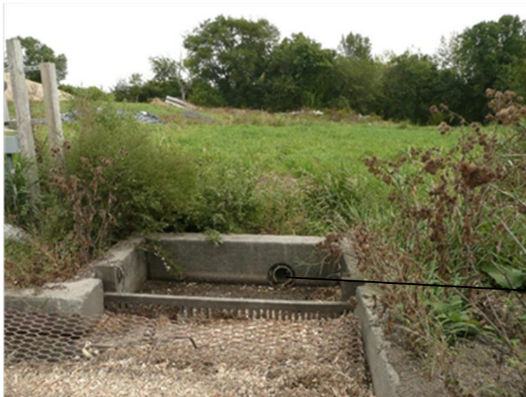
Figure 2: Silage runoff collection point flowing by gravity towards the stream.
