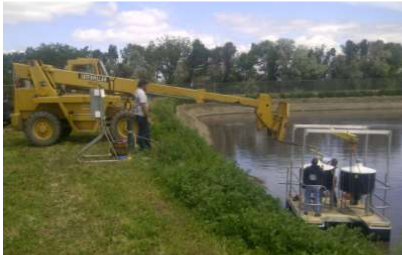
PIC 1 - LOADING WORK BARGE TO SET UNITS IN PLACE ON LAGOON.
