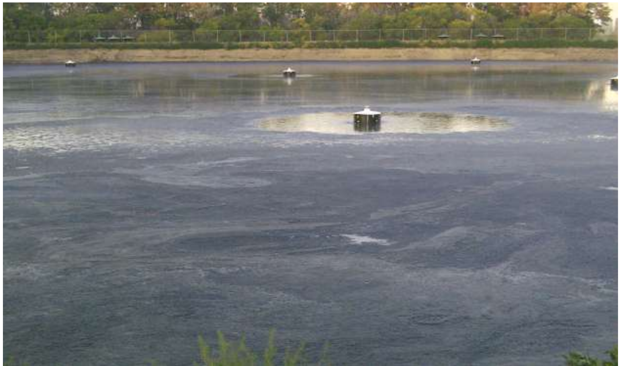
PIC 3 – JUNE 11 TH 2012, SCUM COVERS MOST OF THE LAGOON SURFACE 15 MINUTES AFTER START-UP
