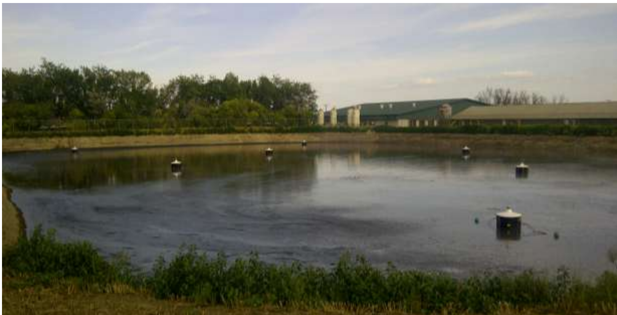
PIC 2 – UNITS SET IN PLACE. NOT YET POWERED UP.
