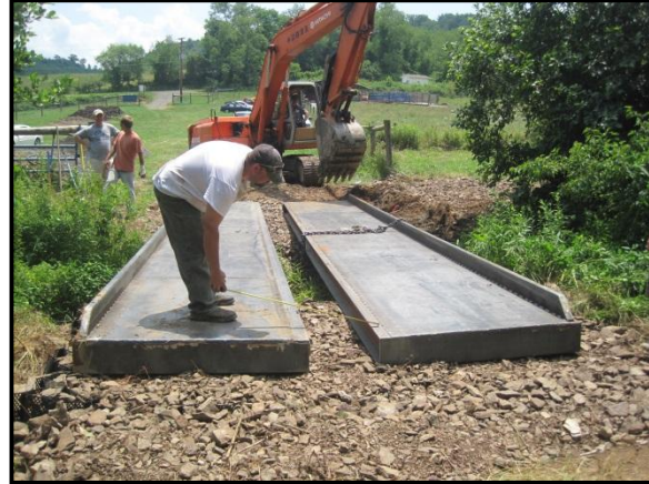
Hillsville, Virginia: Portable timber bridge installation nearing completion.
