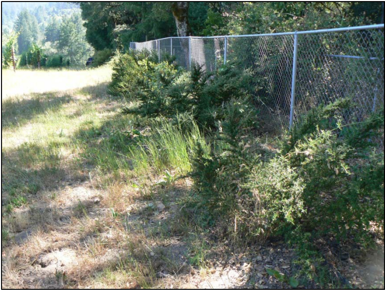
Dierke Enterprises west fenceline 19 June 2012
