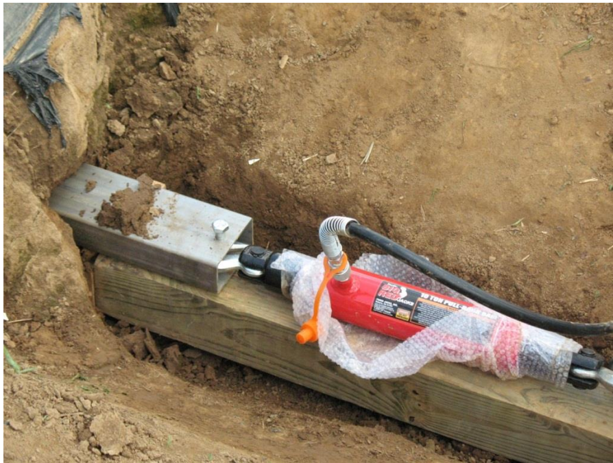
Figure 8: Extraction of Channel Excavator
