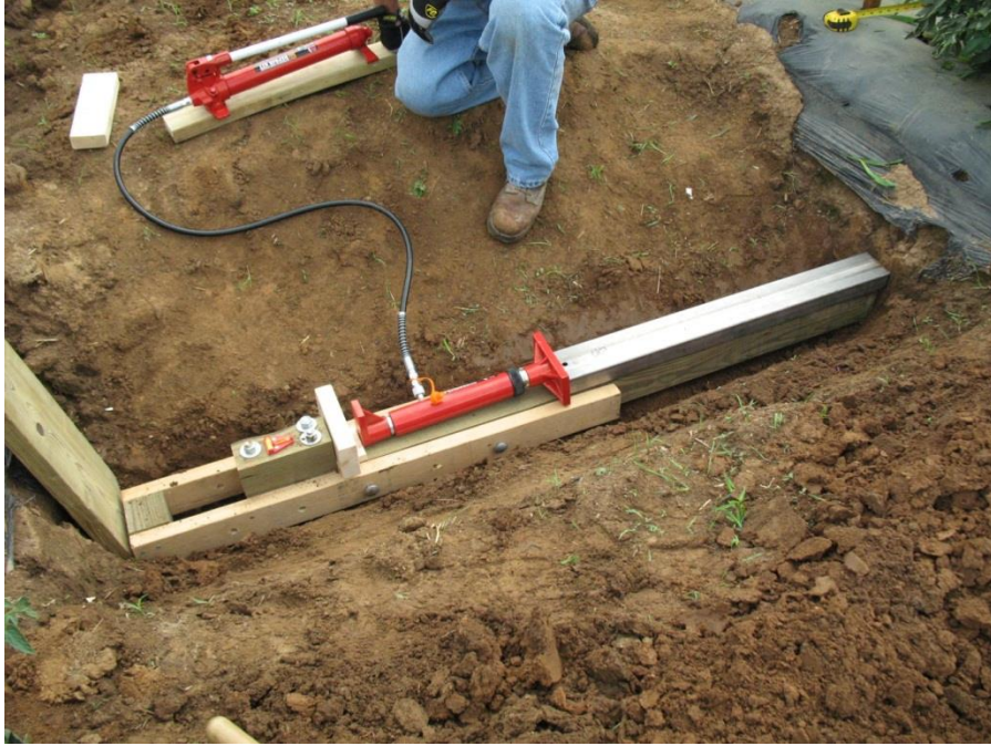
Figure 9: Excavating Pan Channel Being Forced Under Plant Bed by Hydraulic Cylinder/Piston
