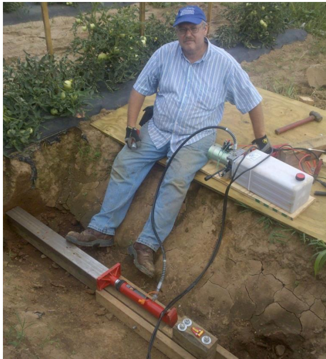
Figure 10: Hydraulic Pump System
