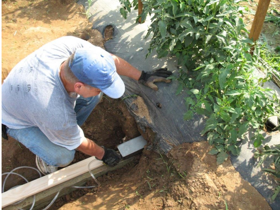
Figure 11: Connecting Drain to Pan
