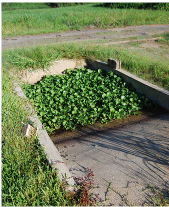
Image 1. Sediment trap box.
