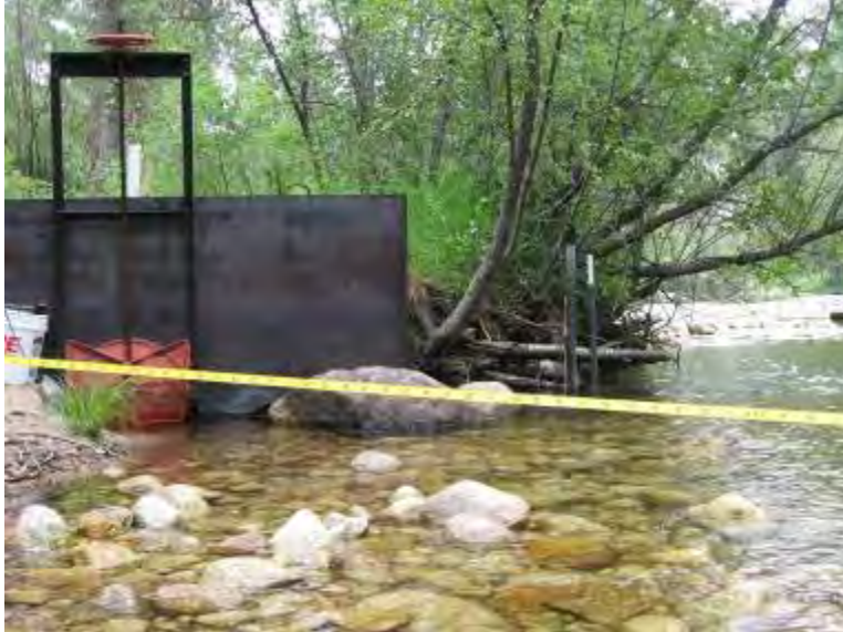
Figure 2. An example of a POD. Pictured is an irrigation headgate with a continuous stage recorder located directly downstream.
