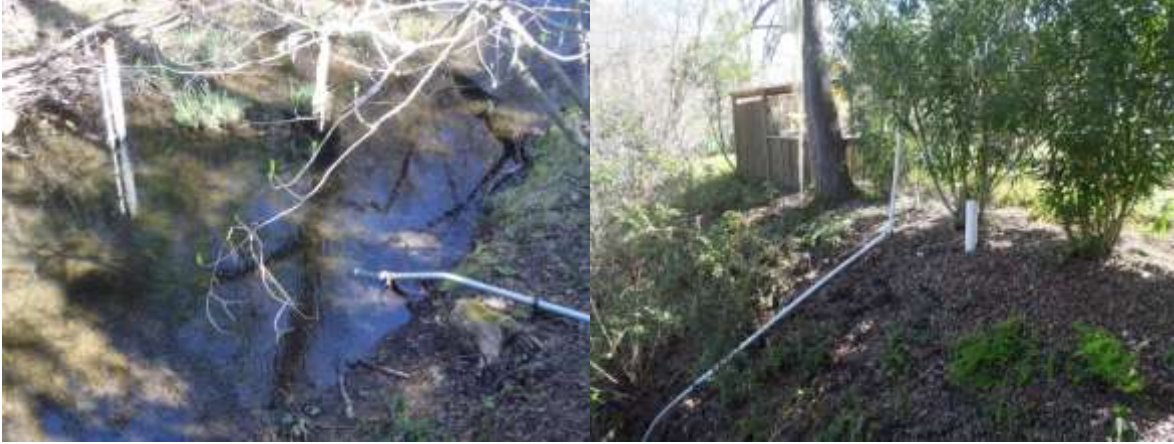
Figure 5a. Global Water gage installed in the McNab Creek Watershed
