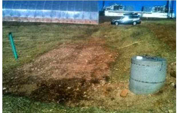
Buried 1500-1600 gal. concrete cistern
