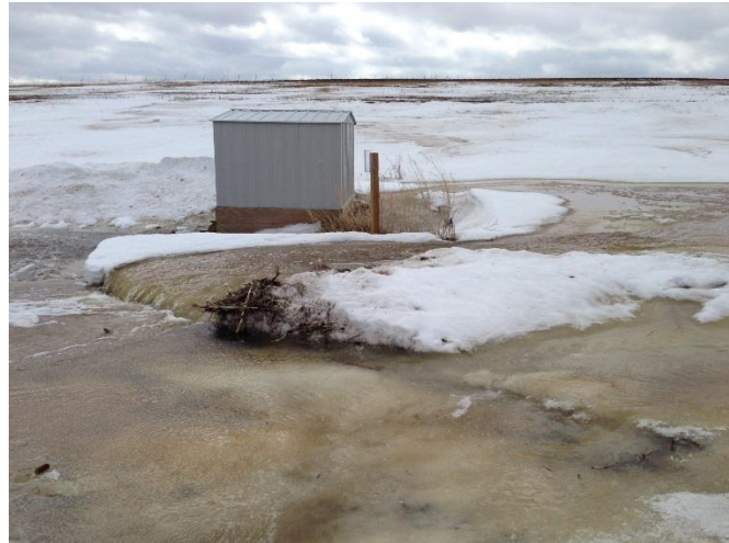
Figure 20. Wisconsin in-line station with bypass
