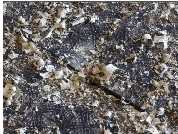
Picture 4. Raised tile edges
