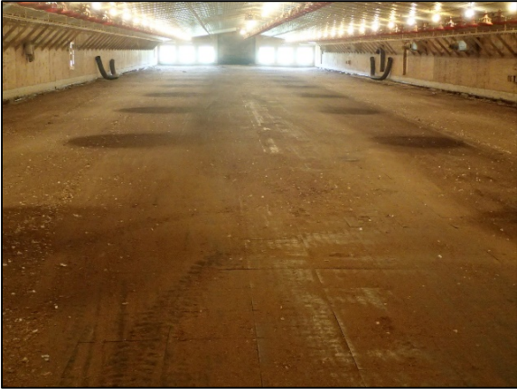
Picture 6. Raised tile edges
