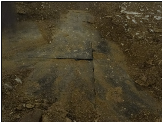
Picture 3. Raised tile edges
