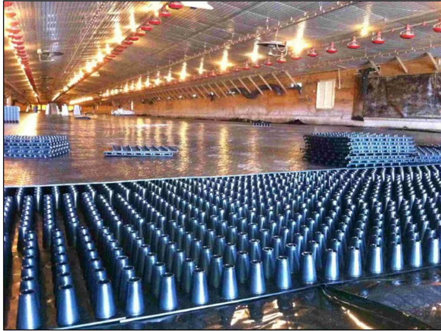
Picture 1. Assembly of the litter-less flooring system (LFS) manufactured by AviHome.
