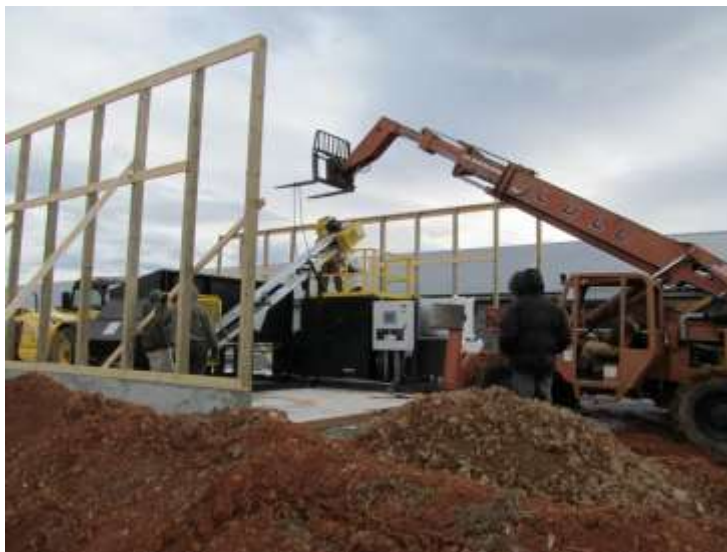
GR unit being set in place on the concrete pad
