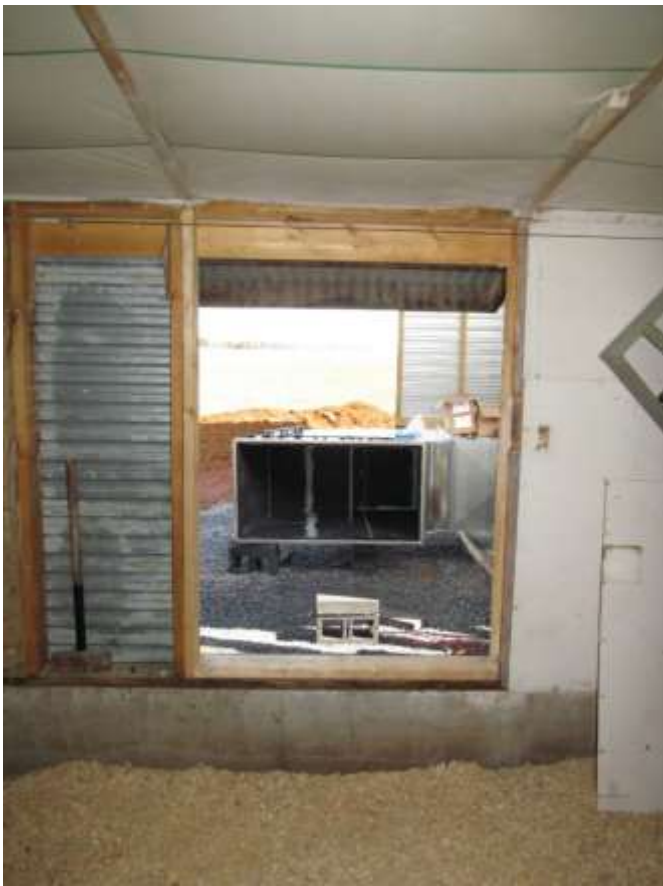
Installation of the duct work into the poultry house
