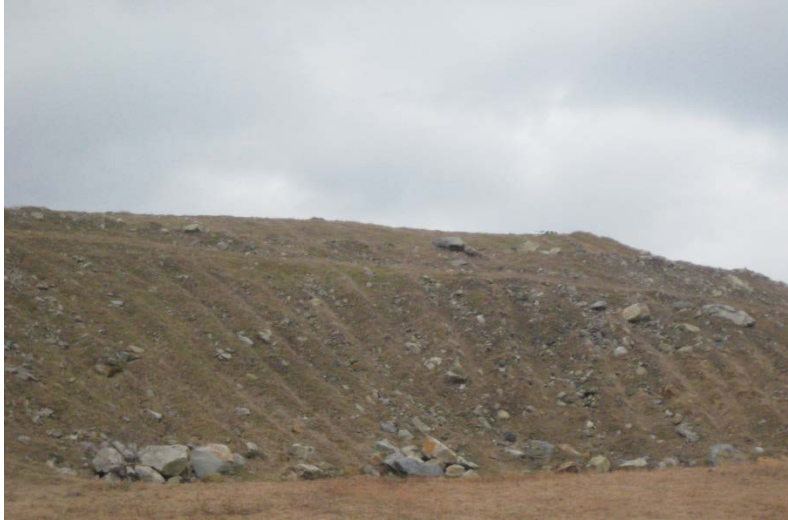
Loosely-graded slopes and reduced ground cover in Kanawha County, WV
