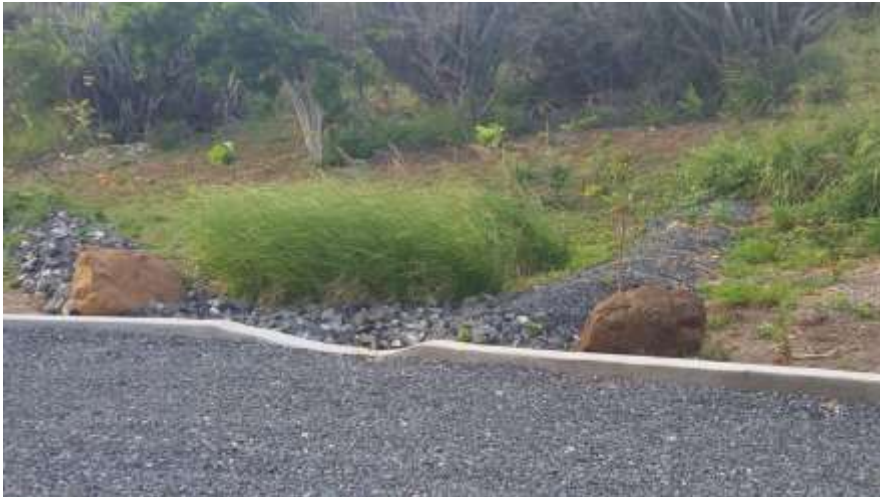
Restoration site in Guanica uses Vetiver grass to slow down water and reduce erosion. Photo: Roberto Viqueira
