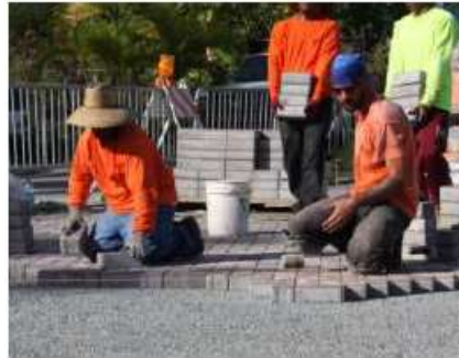
Figure PF15-2. A more complex permeable parking lot retrofit on Oahu.
