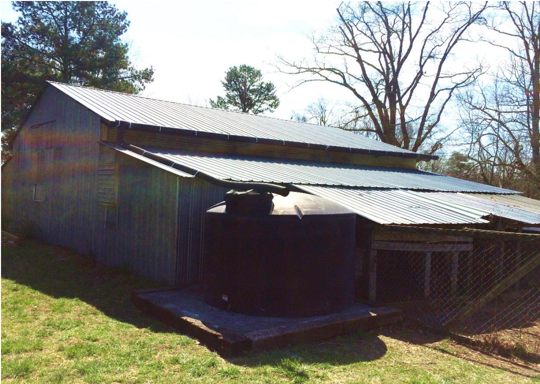
Lee McBride Rain Catch System. Falkville Al. Farm # 3729
