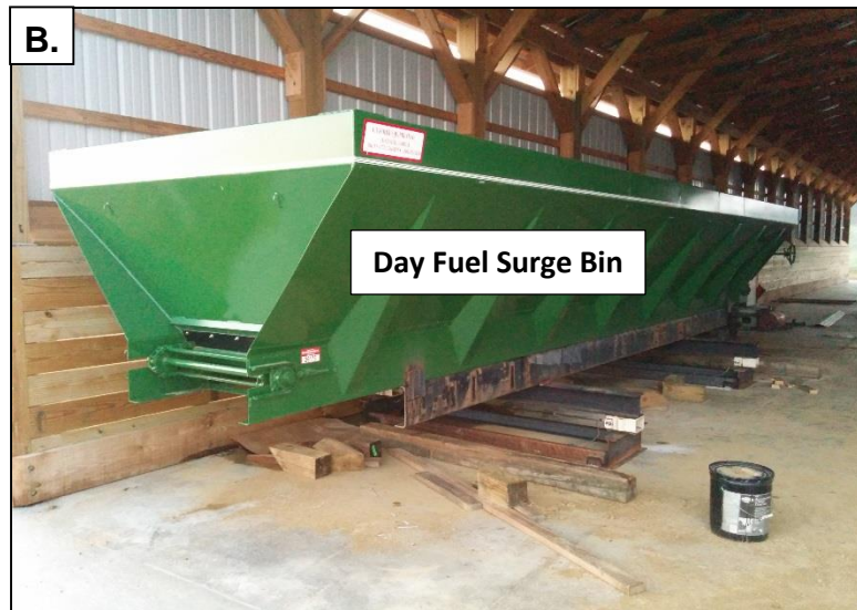
Figure 3. Photographs documenting the fuel storage and conveyance system on the test farm: (A) Fuel conveyor to boiler building; (C) fuel storage building-day fuel surge bin; (C) loading fuel; (D) layout.
