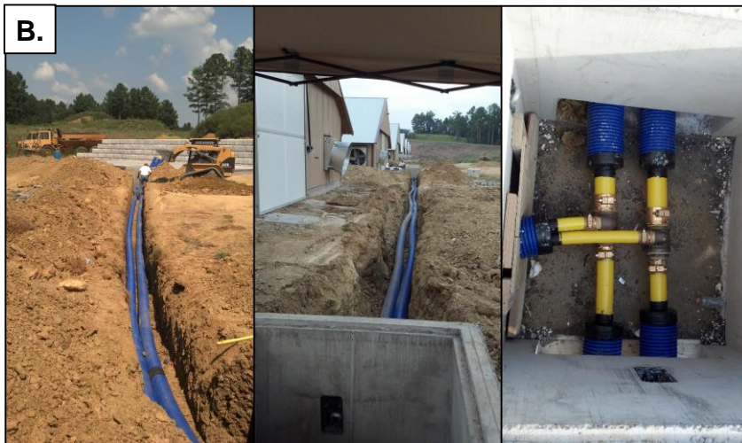
Figure 5. Distribution piping and heat exchanger system for the 100 BHP hydronic boiler at the cooperating test farm: (A) assembling the supply and return distribution piping for production houses 1-4 (right) and 5-8 (left) within the boiler building vault; (B) large diameter pre-insulated PEX hot water supply and cool water return lines from the boiler building (left), between the poultry houses (center), and branch points into the production houses (right); (C) hot water fan coils; (D) 2" schedule 10 hot water supply and return lines within production houses.
