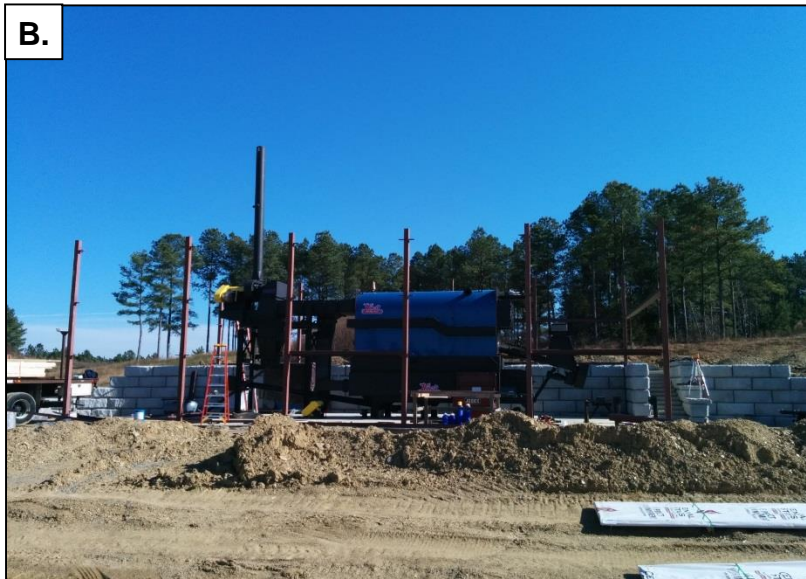
Figure 2. Assembly of 100 BHP hydronic boiler at the cooperating test farm: (A) Crane sitting boiler top; (B) 30x50 ft building being constructed around boiler; (C) assembled boiler close-up; (D) boiler control panel.
