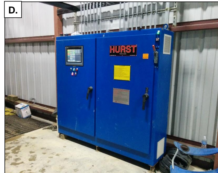
Figure 2. Assembly of 100 BHP hydronic boiler at the cooperating test farm: (A) Crane sitting boiler top; (B) 30x50 ft building being constructed around boiler; (C) assembled boiler close-up; (D) boiler control panel.
