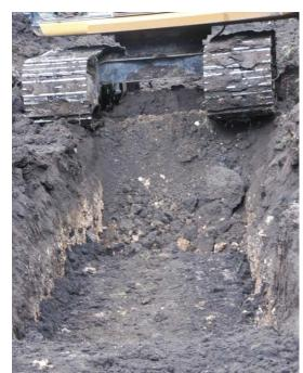
Where the top of the trench meets the bottom of the tank should also consist of at least 18" of compacted clay.
