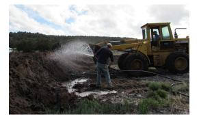
When the clay is the correct consistency, put it back in the newly reconstructed tank in 6" layers ("flights") using the dozer, excavator, and or front-end loader, and then run over it completely, three times, with preferably a heavy rubber-tired piece of equipment (front-end loader or dump truck), to compact that layer.
