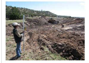
Because the finished tank should have 18"-24" of compacted clay on the bottom, make sure this is accounted
