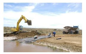
A more focused but elaborate access can be configured by creating a "boat ramp" type approach with geotextile and rock as described above, with the fencing configured to provide access only via the ramp.
