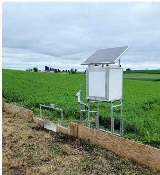
Figure 11. Modified equipment enclosure installed with wingwall and flume.
